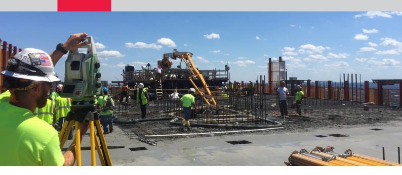
wasn't necessary." Dionisio set GeoMoS to compute an average position of the three building-mounted receivers every 15 minutes, and to average those readings every hour. "So to check for sway, I could compare the coordinates we were using to any past set. Over time, I realized that sway was not an issue on this building and that we could always use the real-time coordinates we had for resections. I observed very subtle movement, but nothing that affected our work or overall building tolerances."
